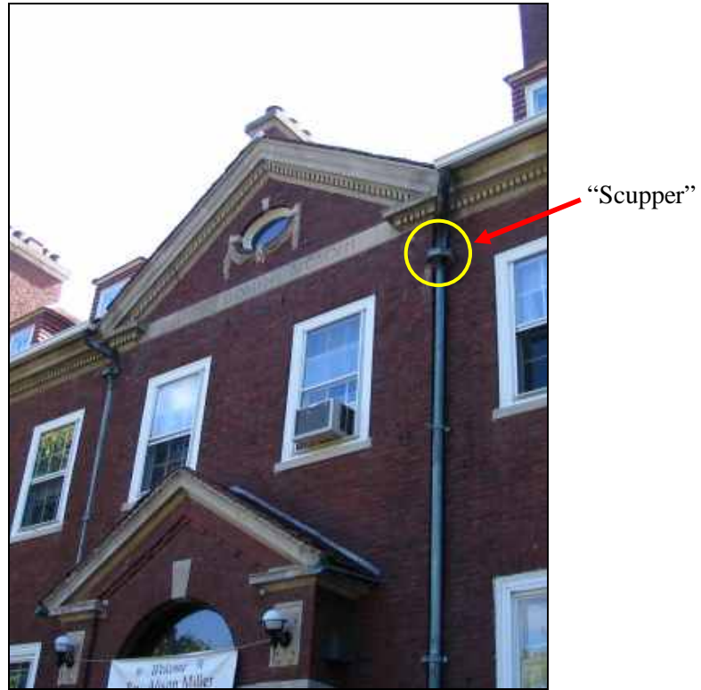
Figure 7 Original Scuppers And Downspouts
